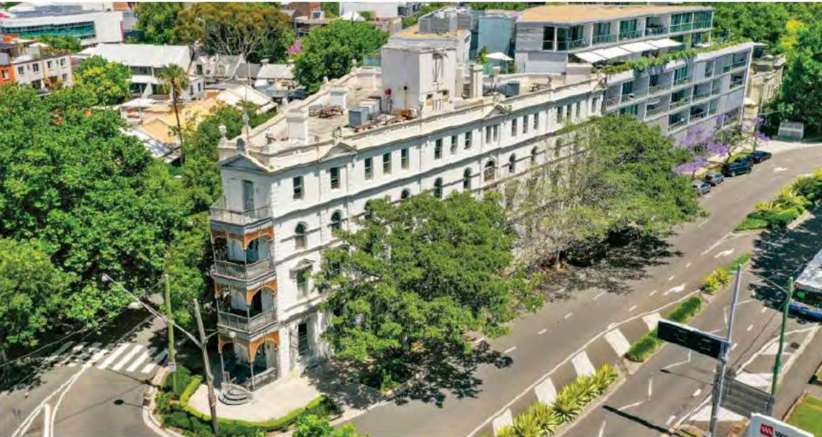
Existing building and rooftop
